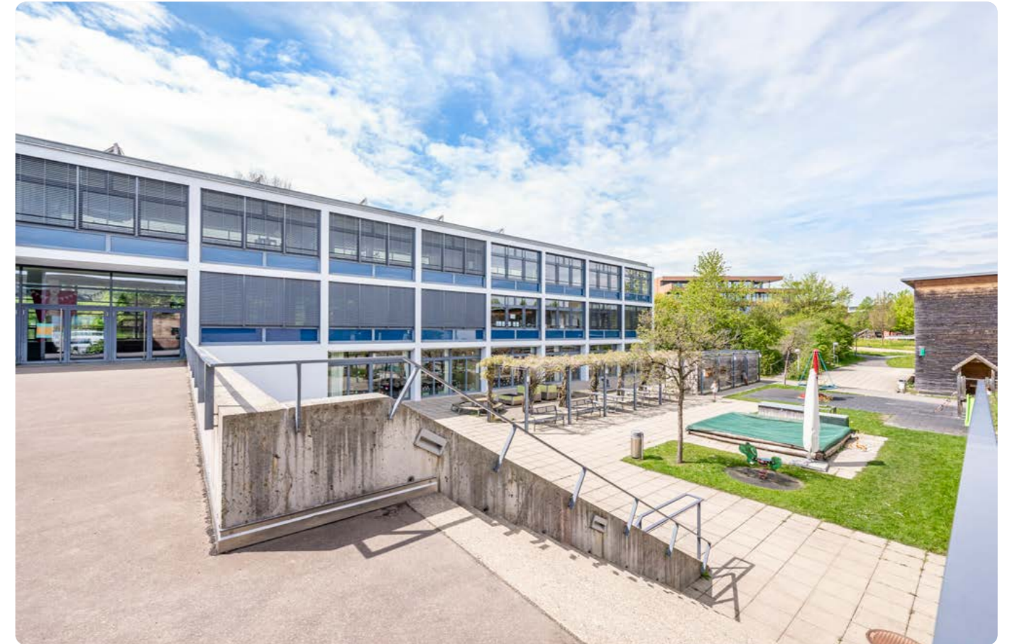
Kemmatten school building with primary school and kindergarten
