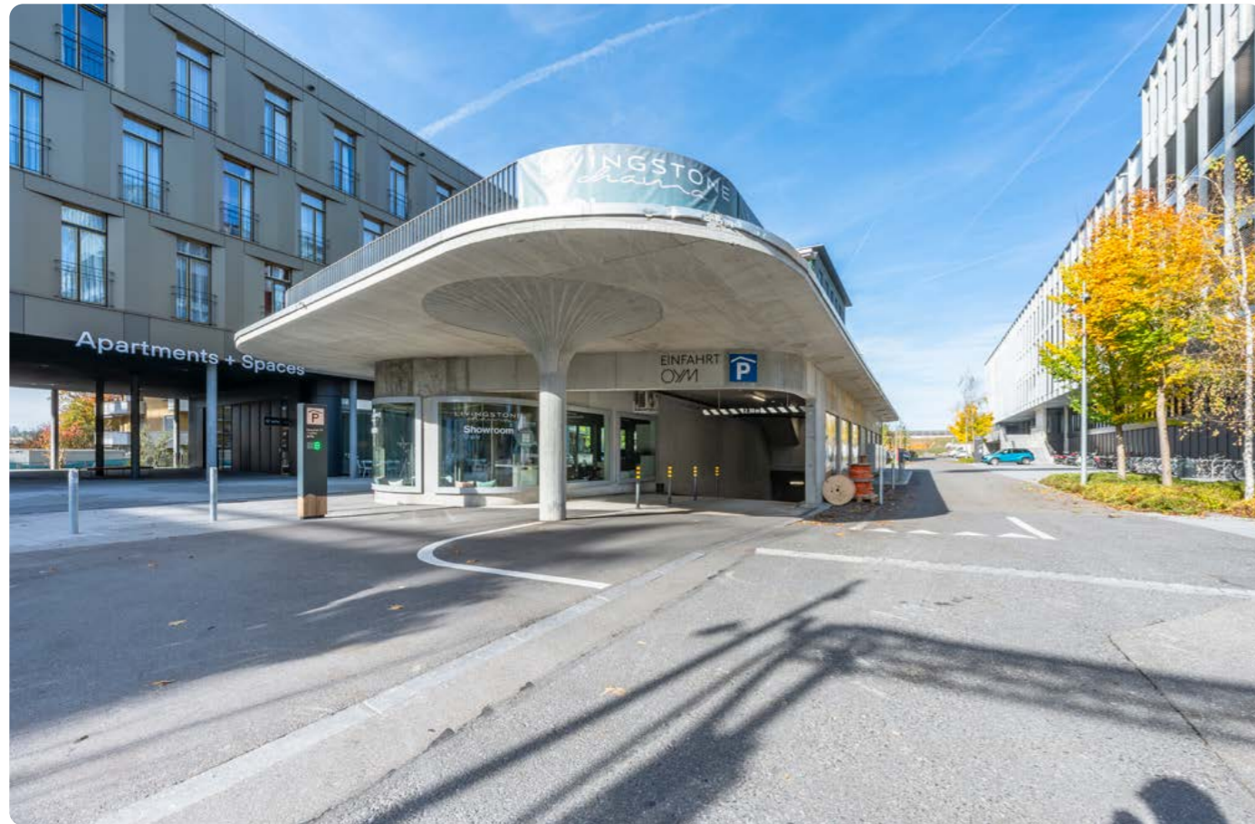
Underground garage entrance
