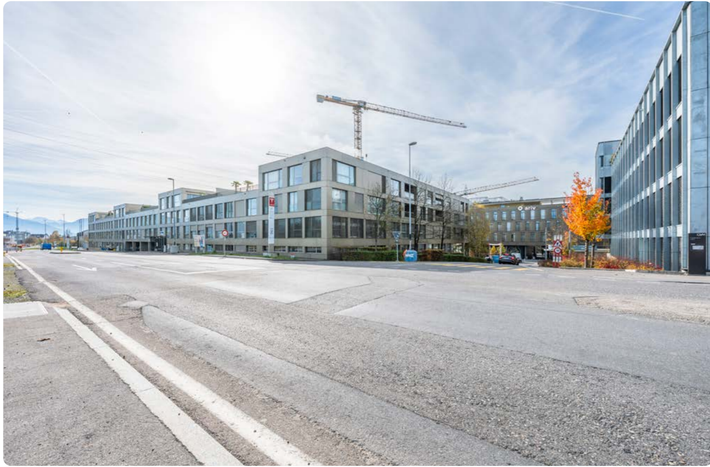
Access via Knonauerstrasse
