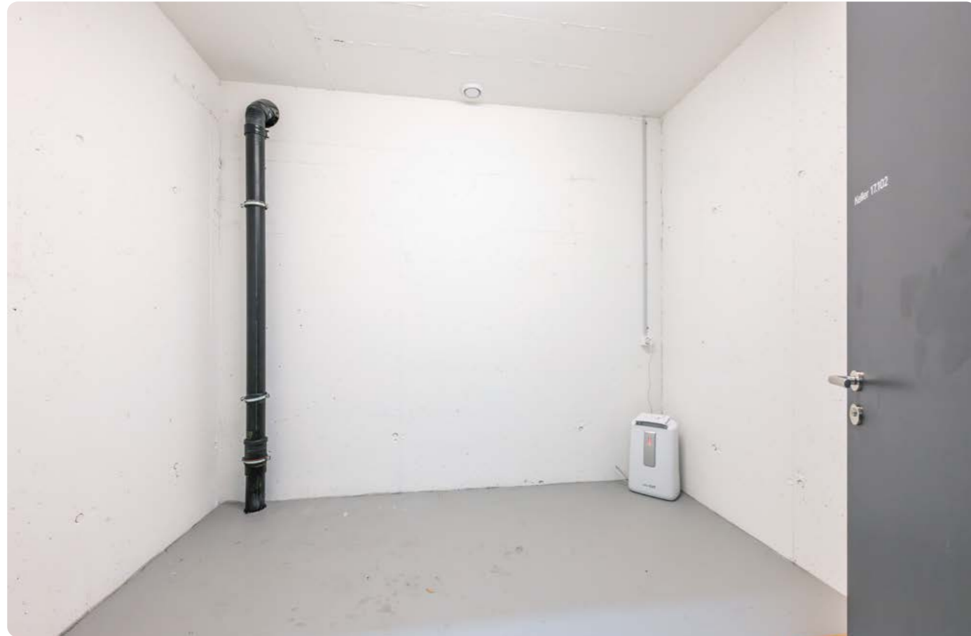
Cellar on the 2 basement level
